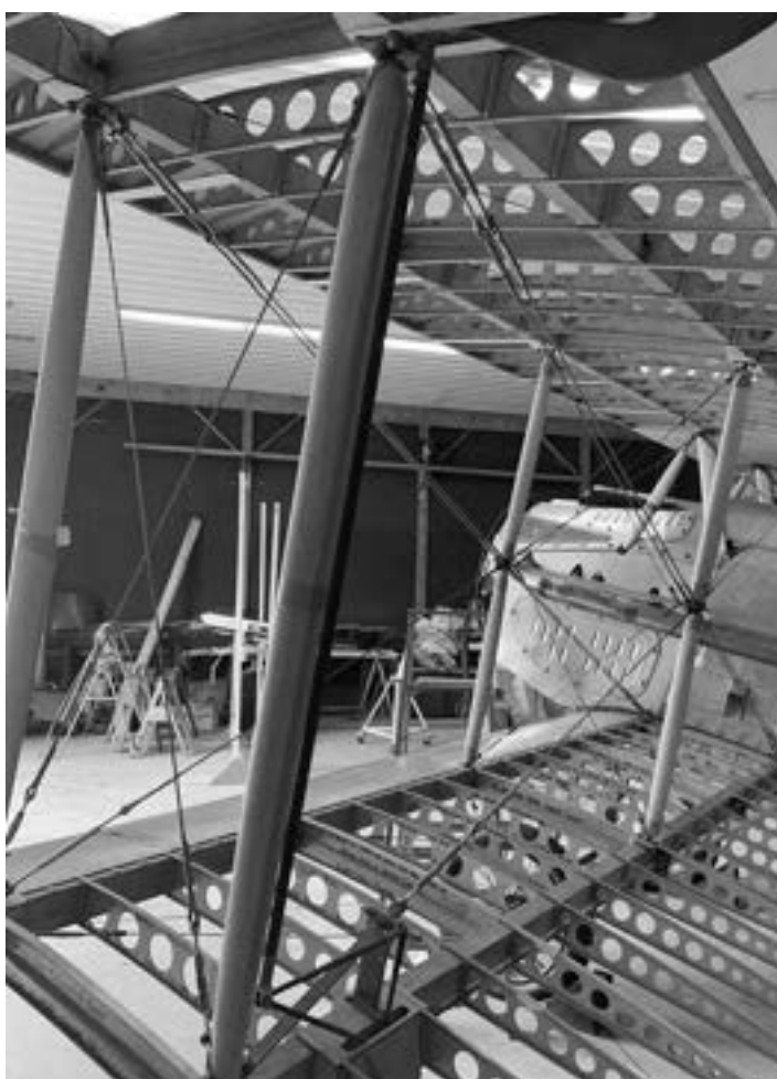
Struts faired in, wing bracing in place and the complicated push-rod activated ailerons are all installed in this photo. With the combination of twin-bay interplane struts, plywood covered leading edges, steel tube struts and steel wire bracing, the SPAD was an enormously strong airplane. If you look closely, you can see individual sponsors names on the wing ribs.
