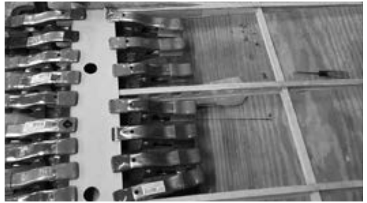
The number of clamps required to glue up the leading edge of the rudders is remarkable. The museum uses a two-part marine epoxy that forms a bond stronger than the material being glued together.
