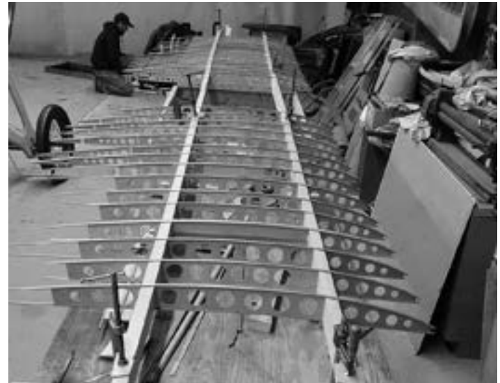
The start of the upper wing. Unlike the lower wings, the upper wing is a 28' single piece wing. The main spars were spliced mid-wing and the wing ribs slid onto them. Keeping the whole structure straight proved to be a challenge.
